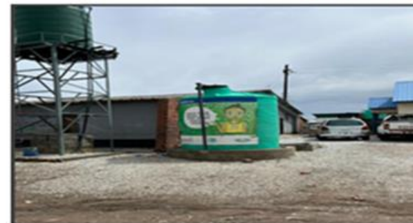
Provision of safe water in Ngwerere
