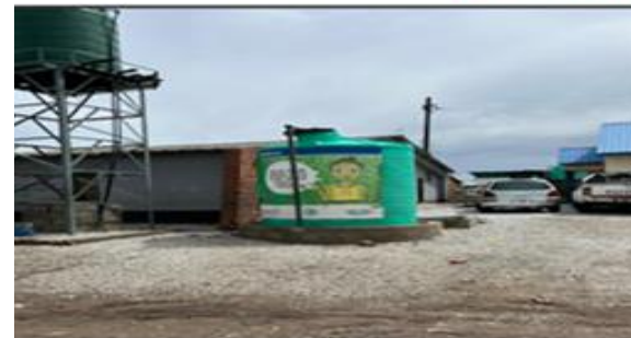
Provision of safe water in Ngwerere
